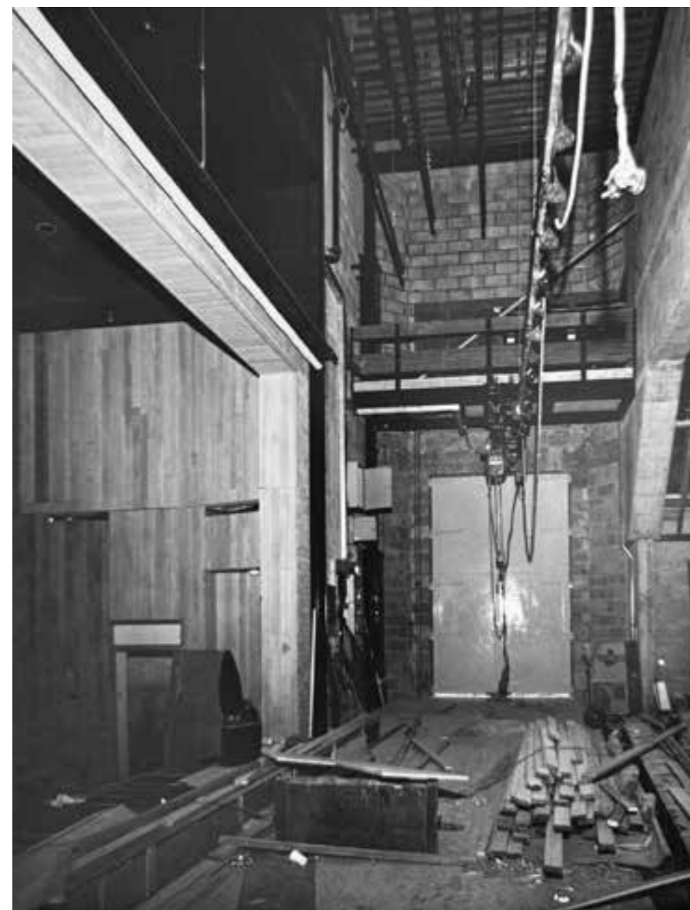
Figure 20: The Stage and flytower nearing completion in 1975 (Source: Leighton Gibbons, 1975)
