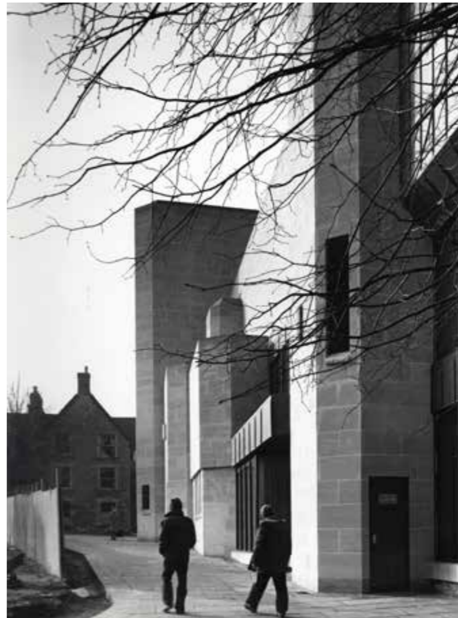
Figure 14: 1975 view of the east elevation of the Theatre viewed from the north east. [Photograph by Leighton Gibbins, from Hopegood Archive]
