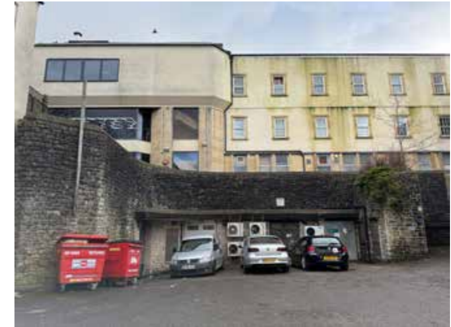
Figure 22: View of the Amulet from the north from Market Place in 2024 showing the c. 2007 mock-Georgian rear facade of Nos. 3-4 Market Place on the right and the north elevation of the Amulet on the left. The jettied committee room on the left has lost its standing seam lead cladding, and the windows were added following planning permission to convert the space into a flat in 2015 (compare with Figure 15 ).
