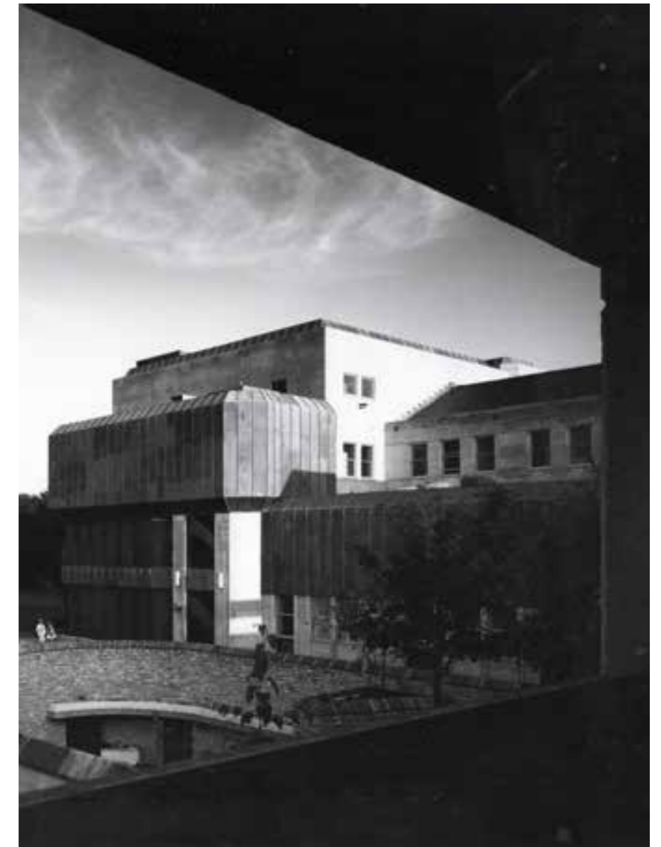
Figure 15: 1975 view of the Theatre viewed from the retirement apartments to the north, showing the lead-clad committee room space on the left, and the north elevation of Nos. 3-4 Market place on the right. [Photograph by Leighton Gibbins, from Hopegood Archive]
