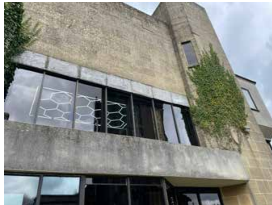
Figure 23: View of the Amulet from the north in 2025, showing the rendered panels where standing seam lead cladding has been removed (compare with Figure 14 ).
