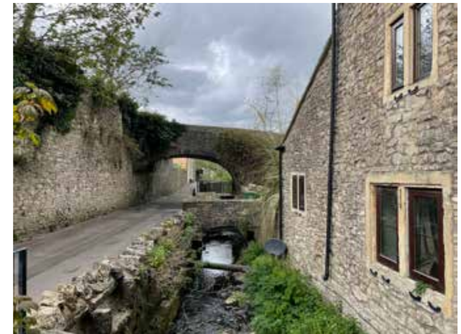
Figure 10: Lower Lane in the steep sided valley to the north of the town, with a Grade II listed bridge over the lane.
