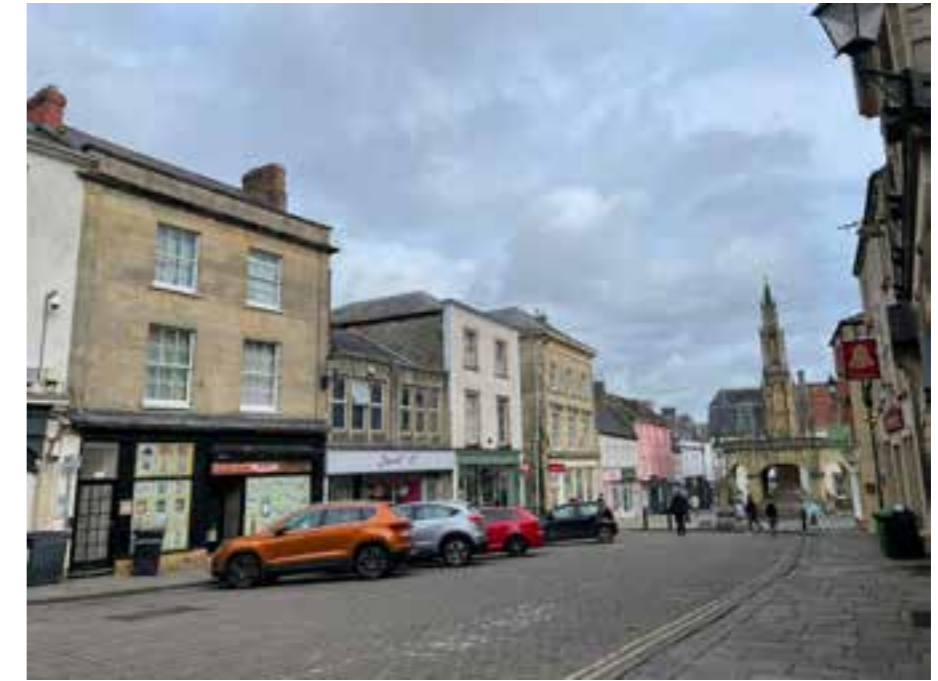
Figure 8: View of the market cross looking north from the High Street
