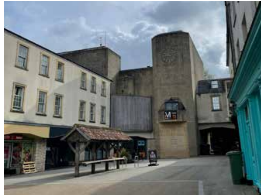
Figure 21: View of the Amulet from Market Place in 2025 showing the c. 2007 mock-Georgian facade of Nos. 3-4 Market Place on the left and the dressing rooms on the right (compare with Figure 13 ).
